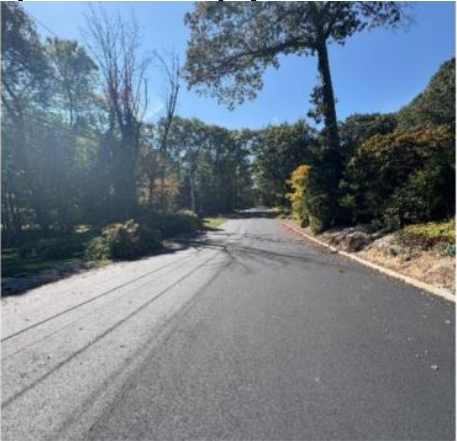
Photo (Left): Livery Road June 2025 image from Google Maps; (Right): Photo September 2025 of rehabilitated Livery Road (Pavement Reclamation)
