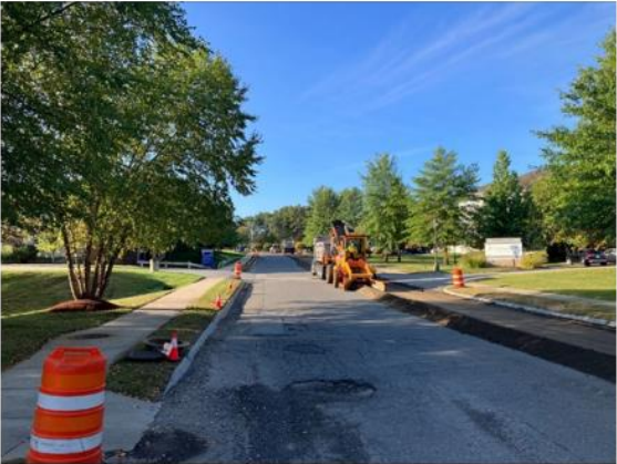
Photo (Left): Research Place September 2025 construction progress photos. Roadway reclamation underway; (Right) October 2025 completion.
